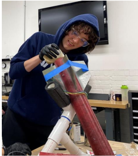
Figure 14: Application of interior fin fillets
